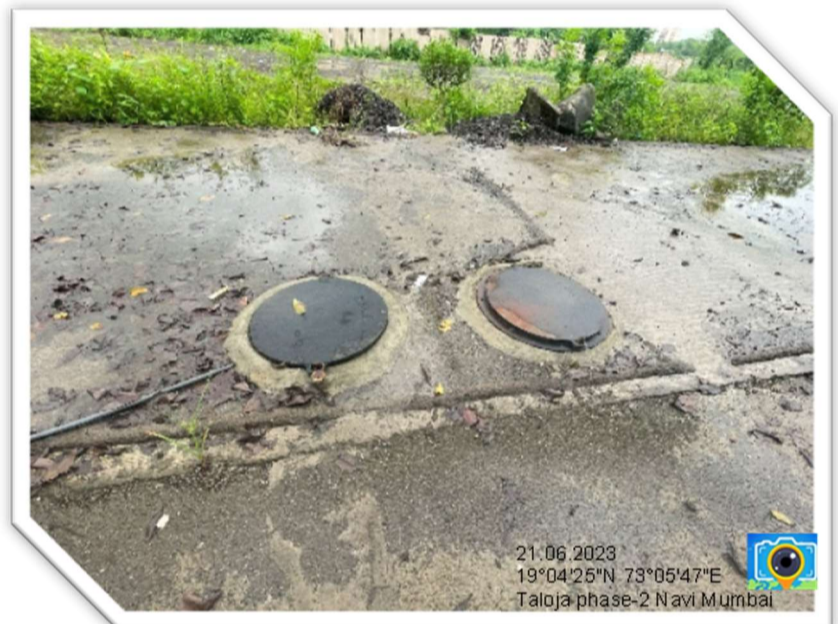
Underground water tanks
